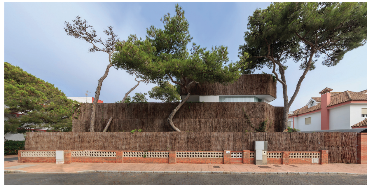
Figure 6. Seaside house in Rota, Cádiz, Spain: south-east elevation. Image: Antonio Luis Martínez Cano, 2015.
